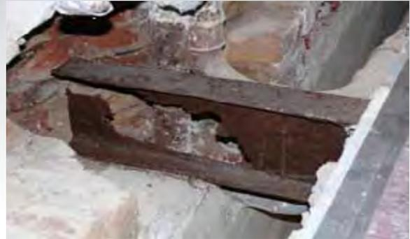
*Failing coatings can lead to serious corrosion and structural failure. In addition to identifying areas that are affected by corrosion, we will develop and recommend repairs to establish structural integrity. As a further step, we can also fabricate the needed plates to reinforce the member or if required, after calculations are performed, replace the support member.*
